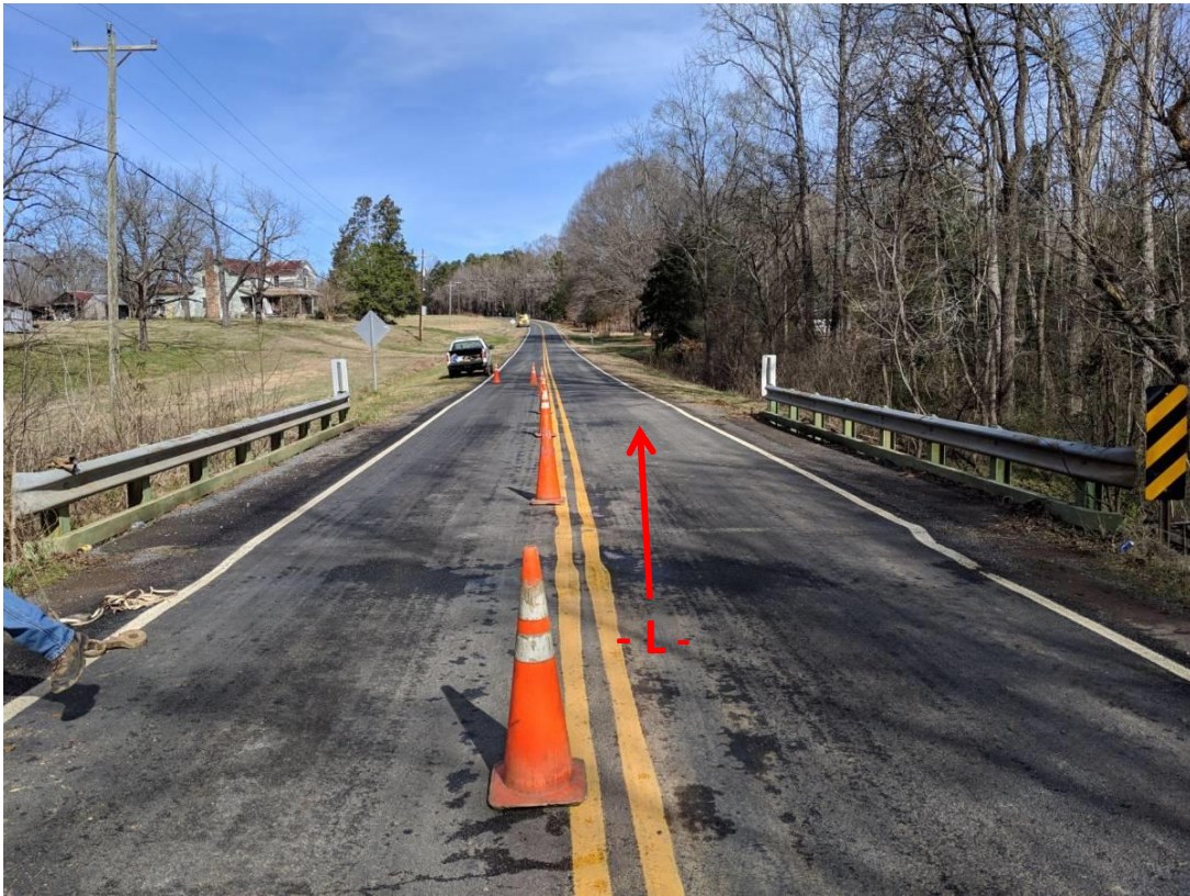
Photograph No. 1: View looking towards EB1 to EB2
