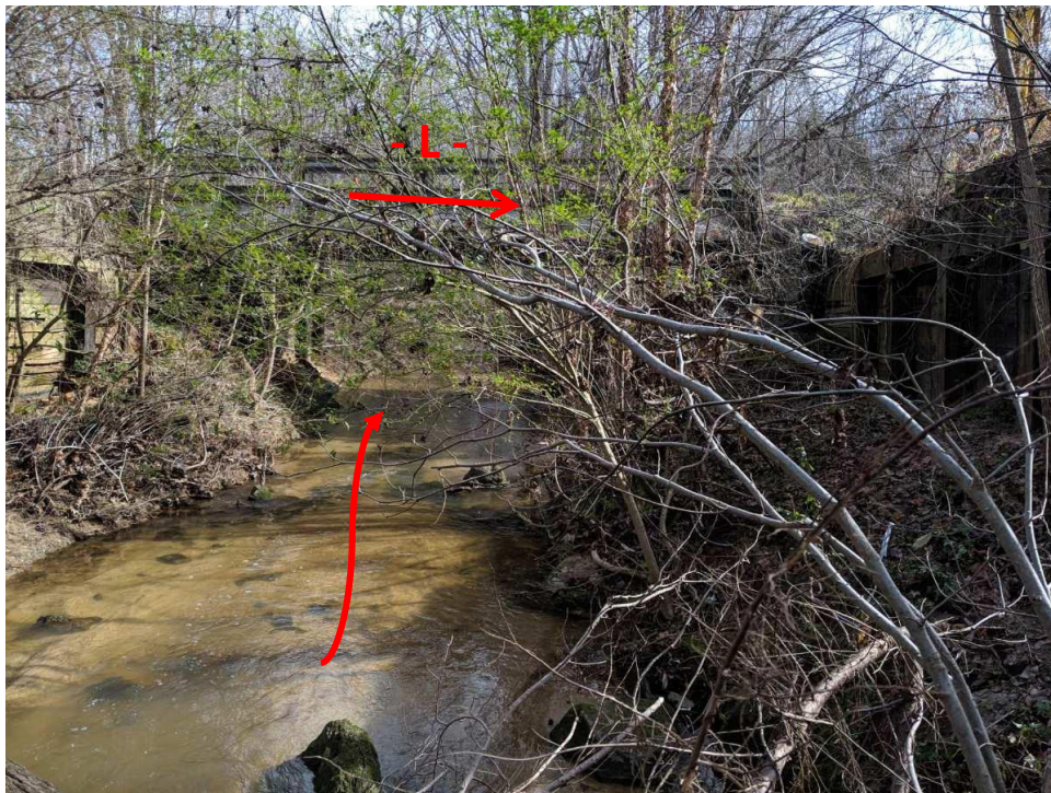
Photograph No. 2: View facing downstream.
